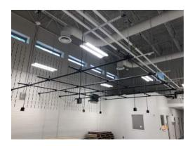
Installation of the Pipe Grid and Drop Down Electrical Outlets in the Aviation Lab 170
